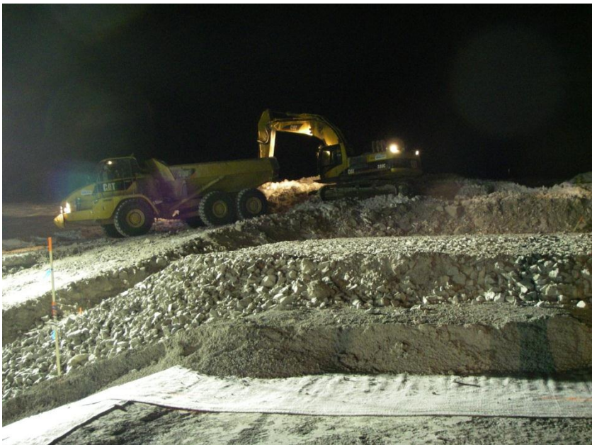
Photo 12: North Dam – Excavator loading snow into a haul truck at the south end of the dam. Photo looking south-east from Station 0+50.
