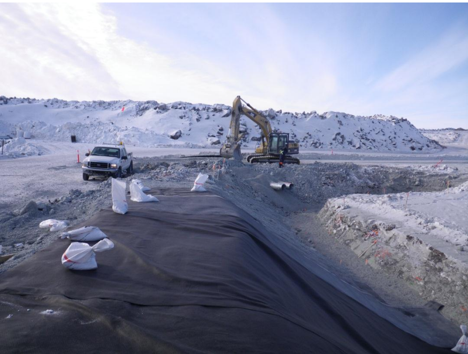
Photo 6: Diversion berm, looking west at culverts installed through the Primary Road.
