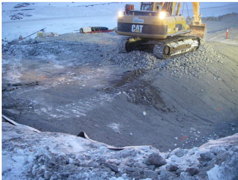
Photo 9: North Dam – Excavator spreading the transition material placed on top of the overliner core. Note the scarred surface of the overliner as a result of excavator traffic.
