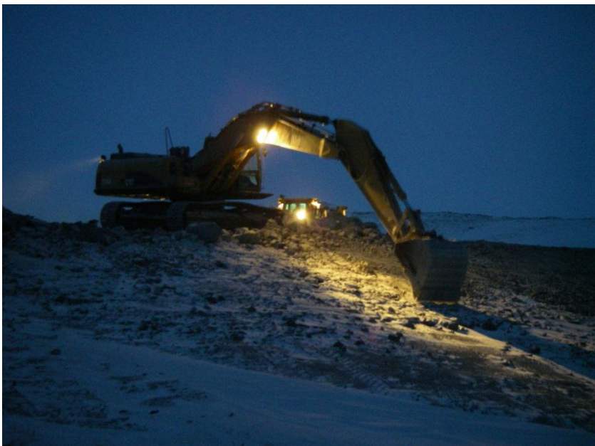
Photo 12: North Dam – Excavator loading snow into a haul truck at the south end of the dam. Photo looking south-east from Station 0+50.
