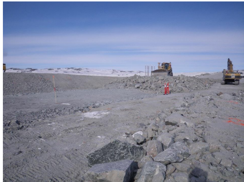
Photo 3: CAT D8 dozer placing ROQ on the north dam. Photo looking north.
