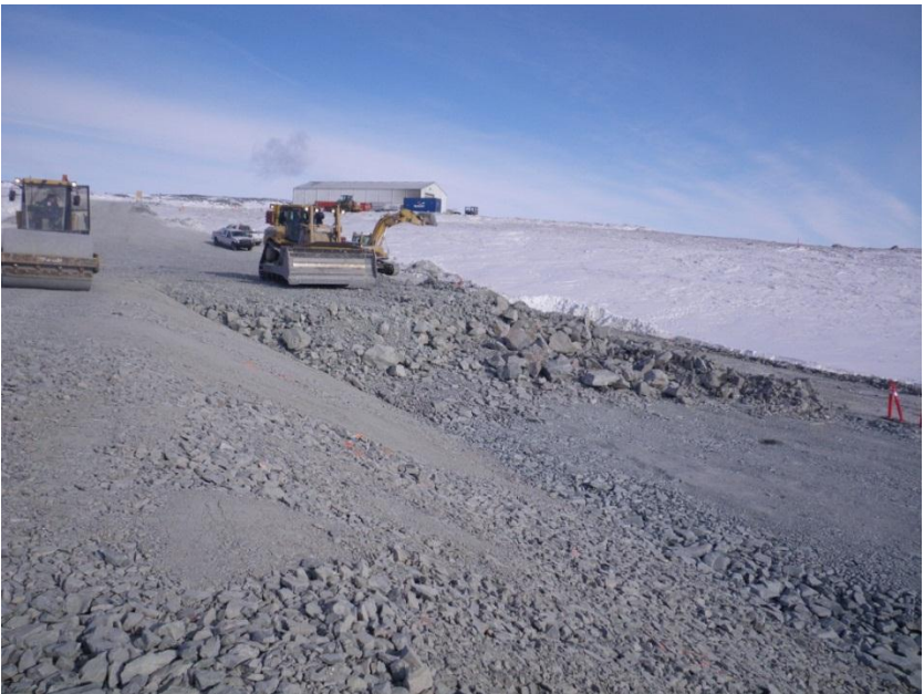
Photo 4: ROQ placement at the north dam. Note the few large pieces in the working face in front of the dozer. These pieces were removed with the CAT 330 excavator.
