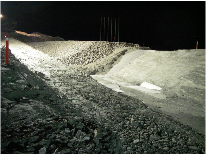
Photo 10: North Dam – south-west view of the completed transition material placement in the south end of the frozen core.
