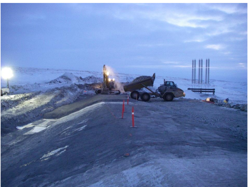
Photo 8: North Dam – Haultruck dumping a load of transition material. Photo looking south-west from about Station. 0+90.
