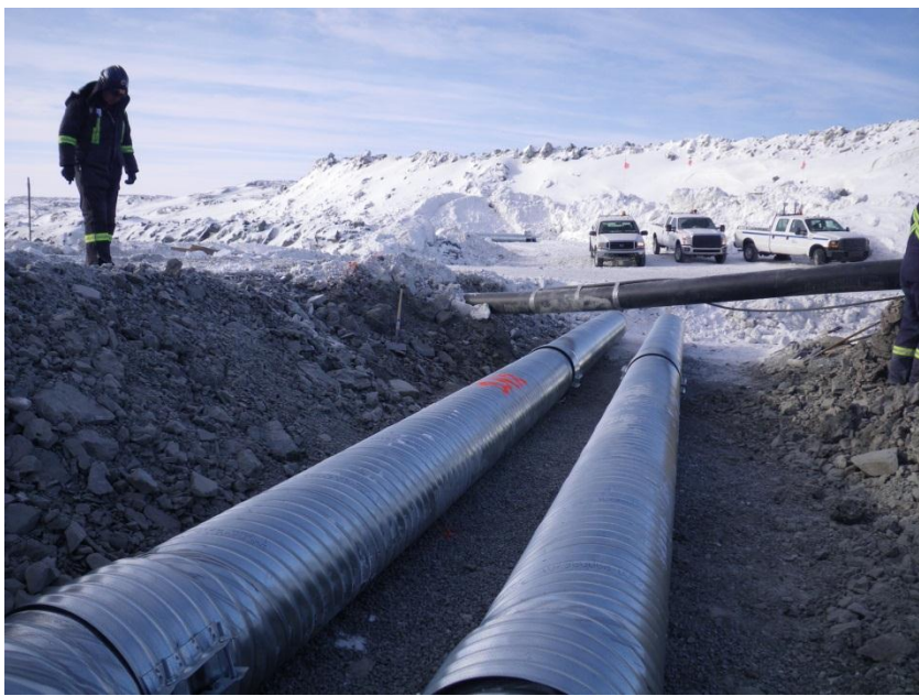
Photo 7: Diversion Berm culverts laid across road, prior to backfilling.
