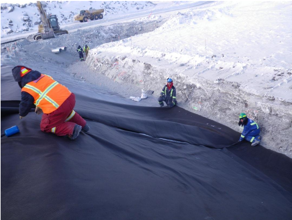
Photo 5: Placement of upper geotextile at the diversion berm/
