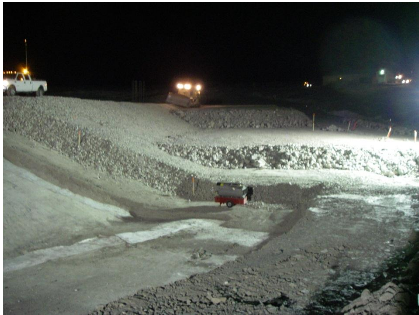
Photo 11: North Dam – progress photo of the second lift of ROQ placed on the upstream side. Note the transition and the first lift of ROQ were stopped around Station 0+90 waiting for completion of the GCL and overliner core placement. Photo looking north from Sta. 0+70
